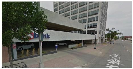
The US Bank parking garage in Sioux Falls, South Dakota, was on the verge of being condemned. Ironhide Construction teamed up with US Bank, McGill Restoration and SDG of Lincoln to devise a plan to save the structure. This included removal of the top deck of concrete, installation of a new deck and concrete, high grade traffic coating system, structural steel restoration at all T-panel connection points, and cleaning and resealing of all the structural site on site.
