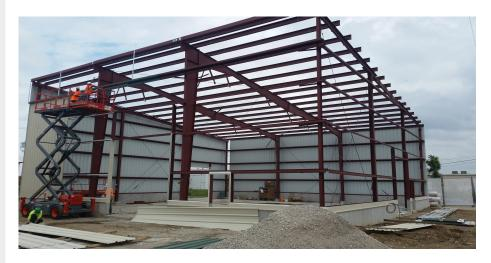
Ironhide Construction erected a 34,520 SF pre-engineered metal building with stucco embossed insulated wall panels and architectural standing seam roof with a large cupola and two-offshoot buildings.
