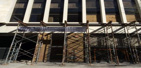
The south precast concrete panel wall of the US Bank parking structure was impacted and began falling off the building. Ironhide Construction was called in to inspect the site. By Noon the next day, the street was shut down, engineers visited and designed a shoring tower to prevent the panels from falling off. The city officials, the Lincoln Fire Department, and Lincoln Police all visited the site in case of catastrophic failure.
