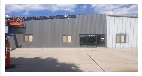
This Parpart project consisted of replacing standard grade panels with 24 gauge 7.2 panel and 24 gauge Masterline 16 on a 6,000 square foot building. Ironhide enjoyed working with the owners and building a relationship throughout this project.
